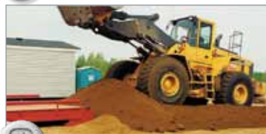
3 Backfill to bulkheads and finish ramps.
