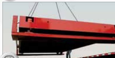
2 Unload and set modules.
